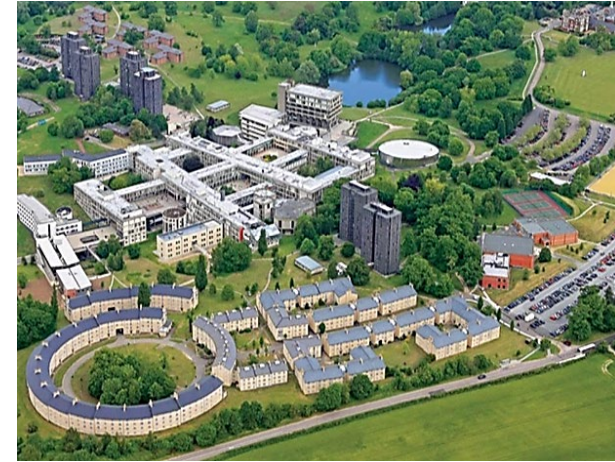
Hospital, Industrial Estate, Campus
